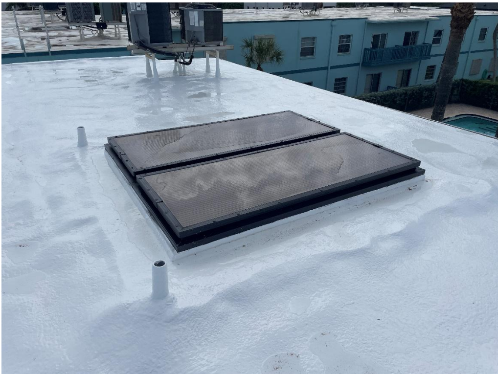
Photos of the recently installed Spray Polyurethane Foam roof with silicone coating, and new skylights.
