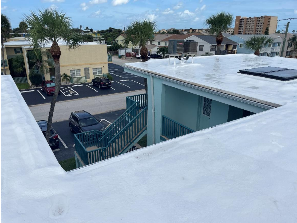
Photos of the recently installed Spray Polyurethane Foam roof with silicone coating, and new skylights.
