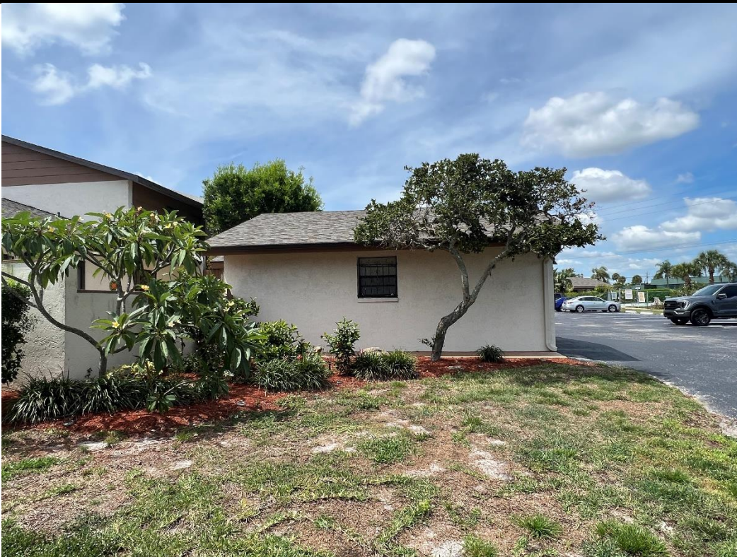
VIEW OF A TYPICAL GARAGE BUILDING
