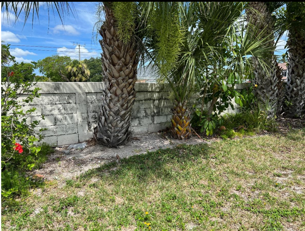
VIEW OF PERIMETER WALL
