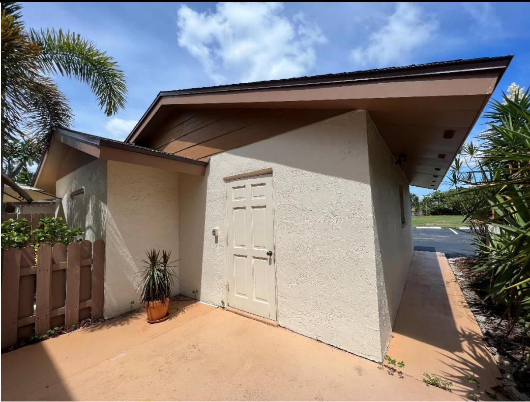
VIEW OF A TYPICAL GARAGE BUILDING
