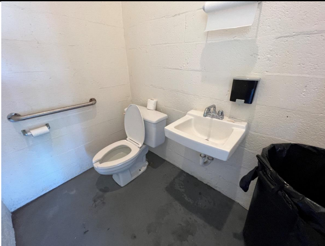
INTERIOR VIEW OF POOL HOUSE
