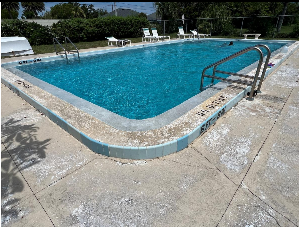
VIEW OF SWIMMING POOL
