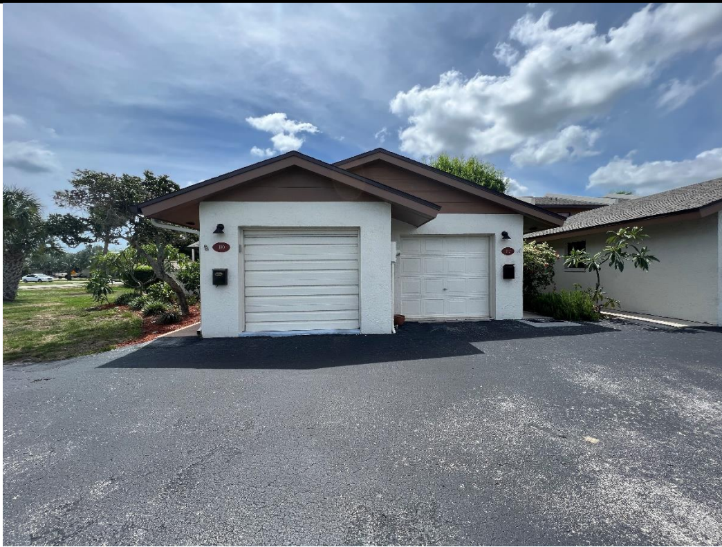
VIEW OF A TYPICAL GARAGE BUILDING
