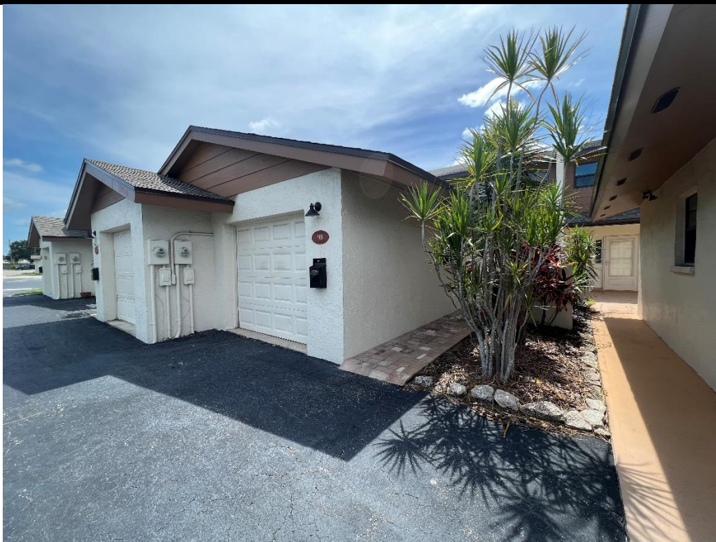
VIEW OF A TYPICAL GARAGE BUILDING
