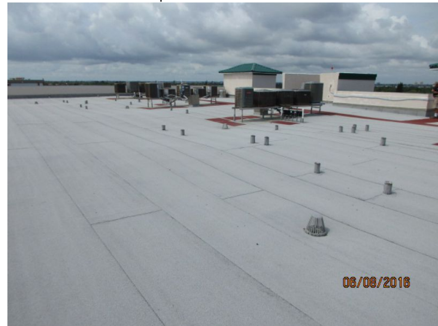
Built-Up/Rolled Asphalt Roof Covering
