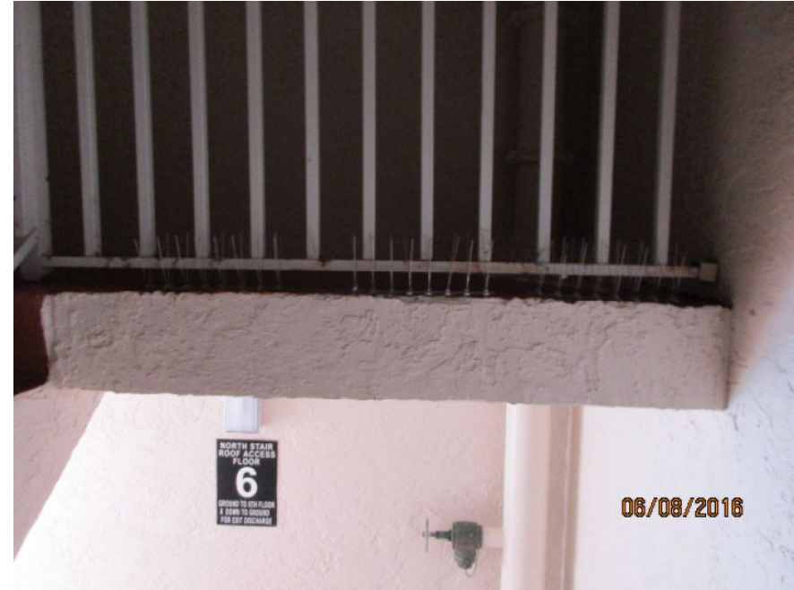
Reinforced Concrete Roof Deck
