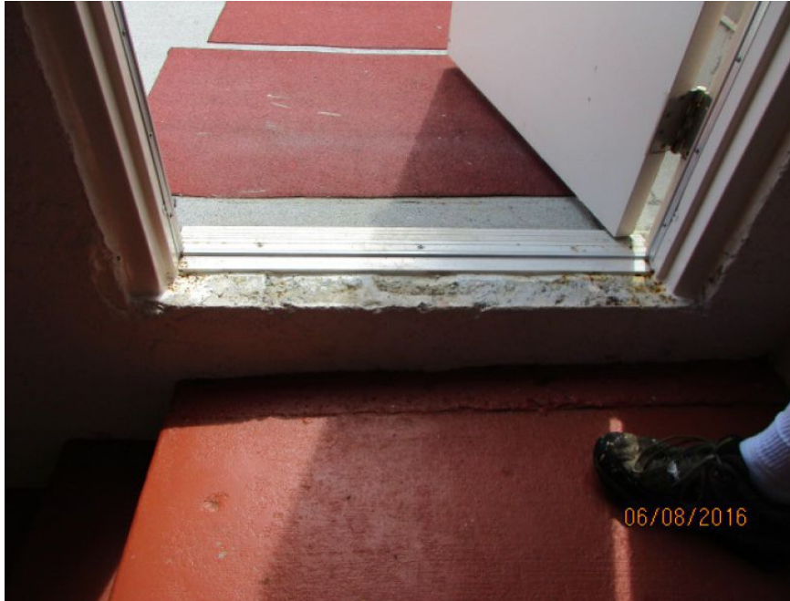
Reinforced Concrete Roof Deck
