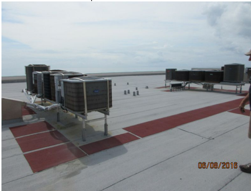
Built-Up/Rolled Asphalt Roof Covering
