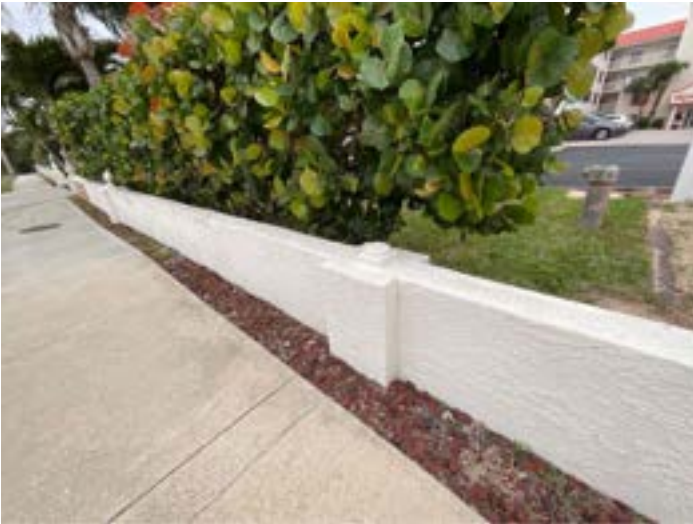
Front of property block wall (east side) - 290'
