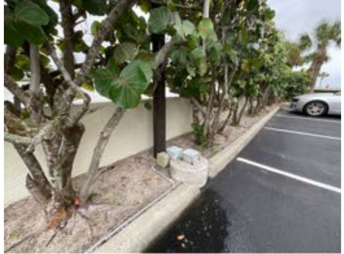
North and south sides of property block wall
