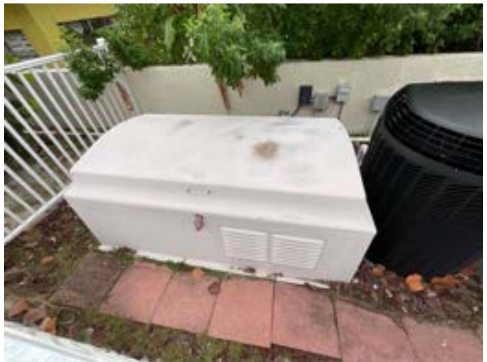
Pool equipment - 2 total
