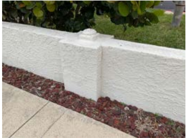
Front of property block wall (east side)
