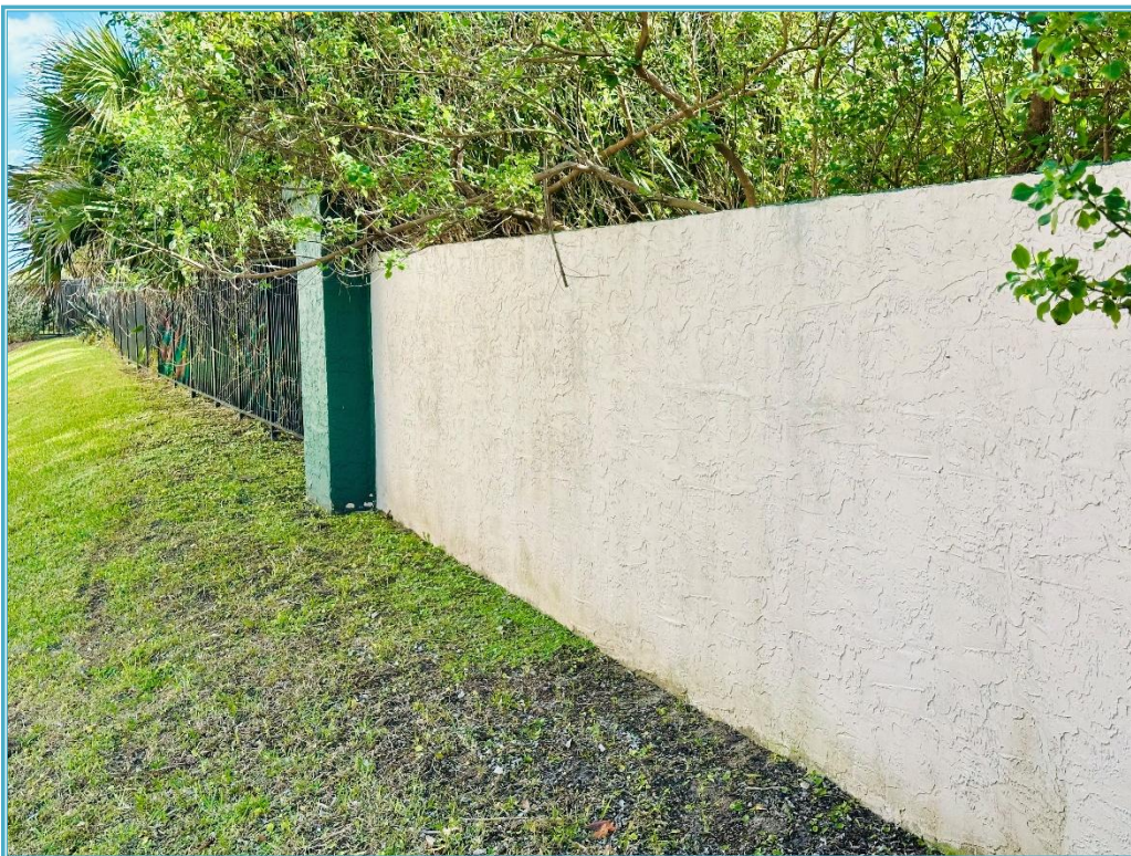
SOUTH PERIMETER WALL AND FENCE
