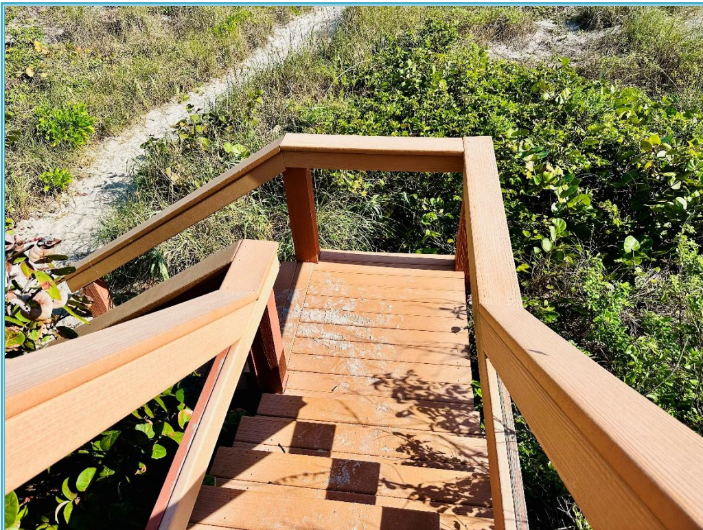
DUNE CROSSING STAIRS
