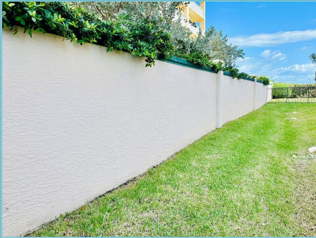
NORTH PERIMETER WALL
