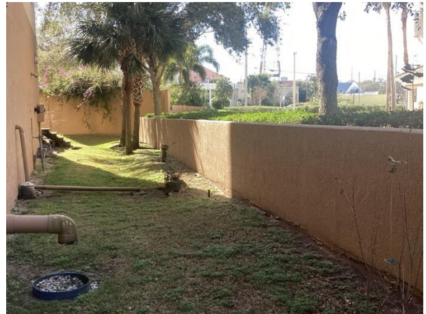
Perimeter wall stucco wall finishes
