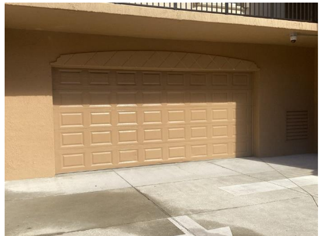
Rear entrance garage door
