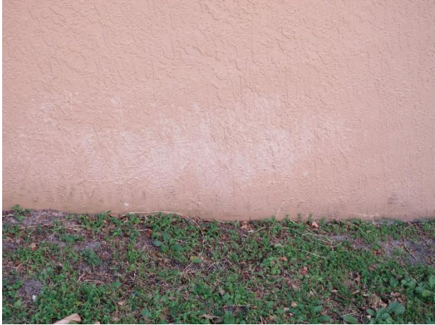
Finish deterioration
