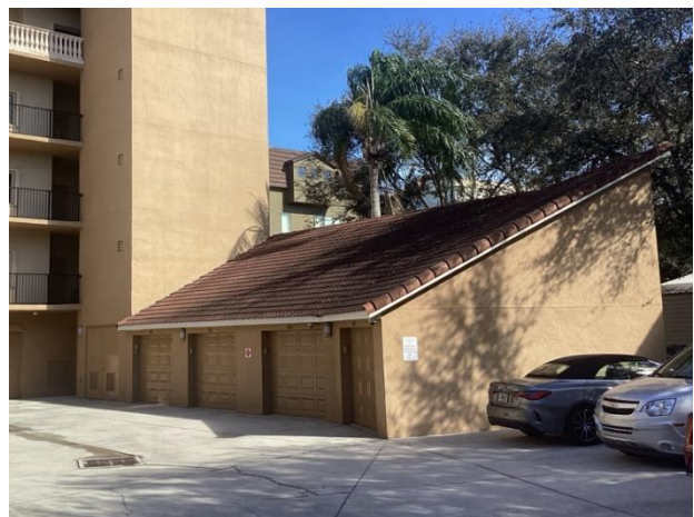
Single garages at the rear elevation
