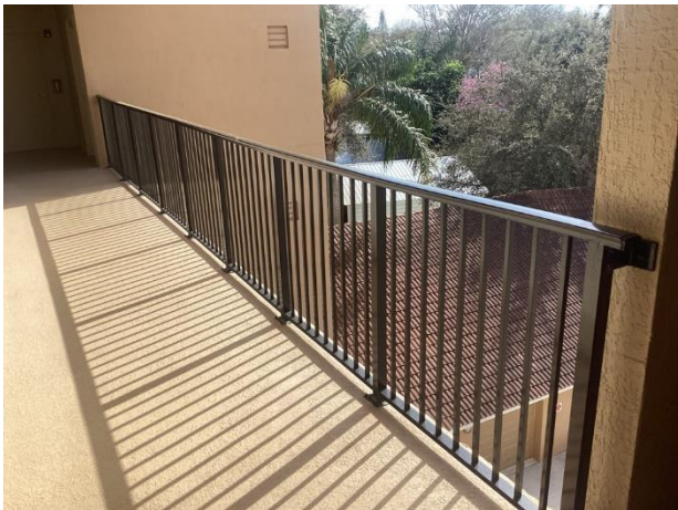
Metal breezeway railings overview
