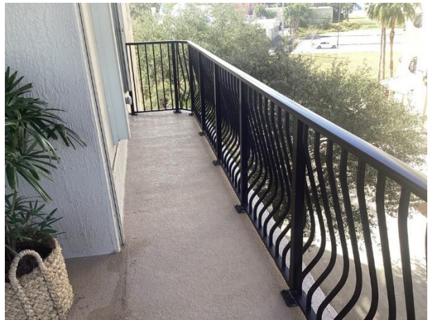
Concrete balcony overview
