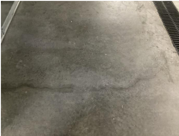
Concrete cracks
