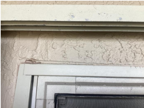
Sealant deterioration
