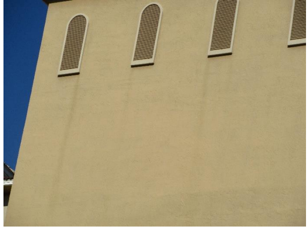
Finish deterioration
