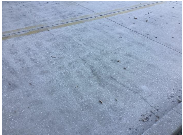
Concrete cracks
