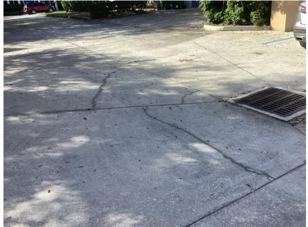
Concrete cracks
