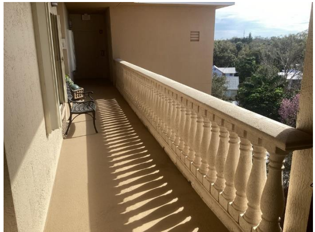
Concrete breezeway overview
