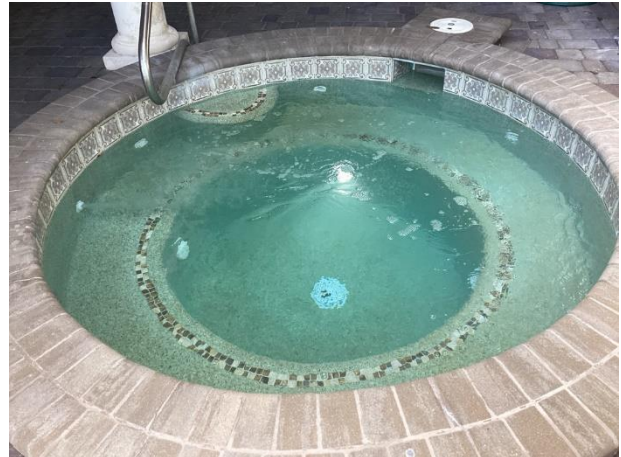
Spa plaster overview
