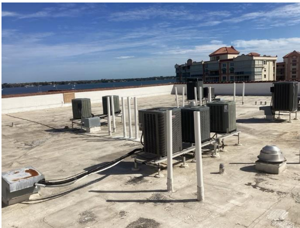
Thermoplastic roof overview
