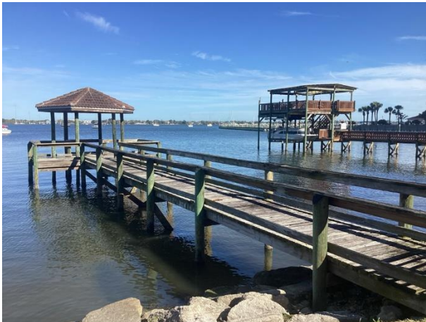
Dock with wood decking
