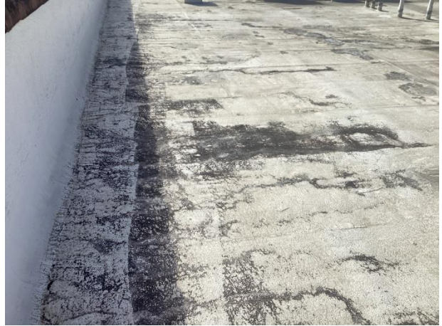
Coating deterioration
