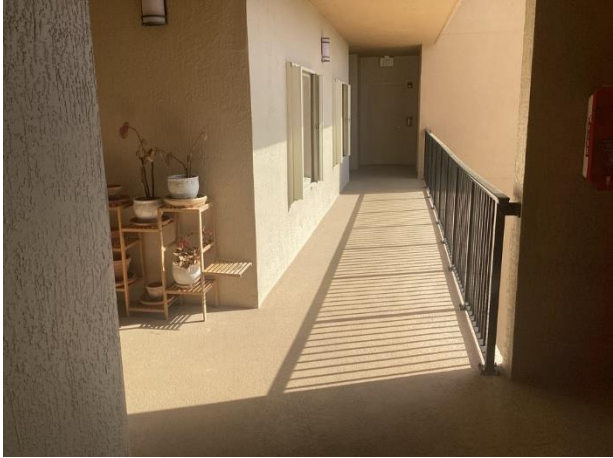
Concrete breezeway overview
