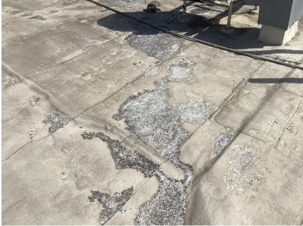
Coating deterioration
