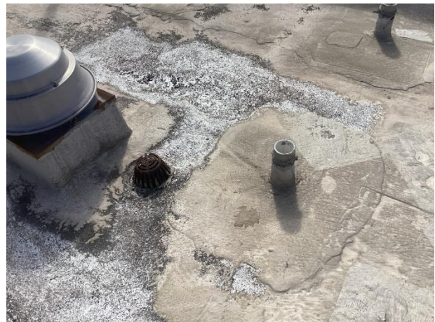
Typical roof drain and penetration
