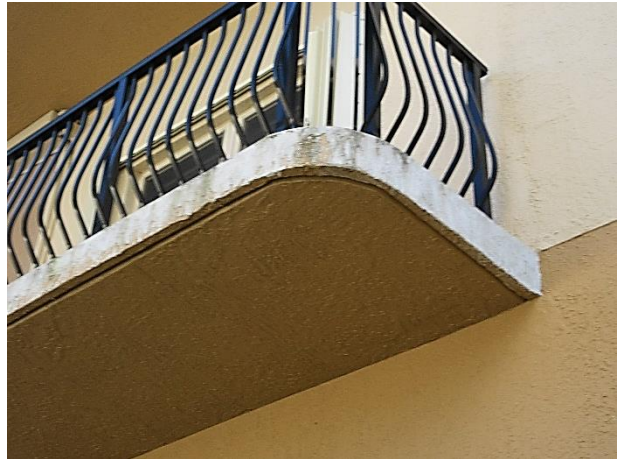
Finish deterioration
