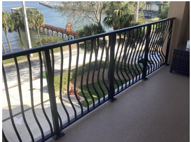
Metal balcony railings overview
