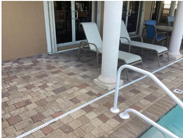
Paver pool deck overview
