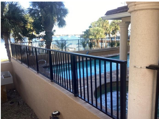
Metal pool railings overview
