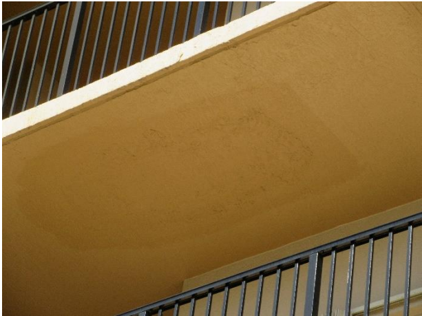
Finish deterioration
