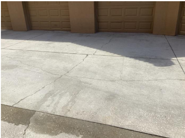
Concrete cracks
