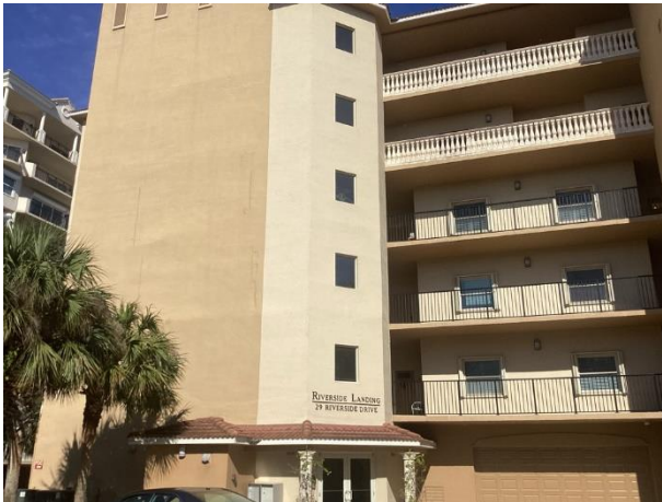
Stucco perimeter wall overview
