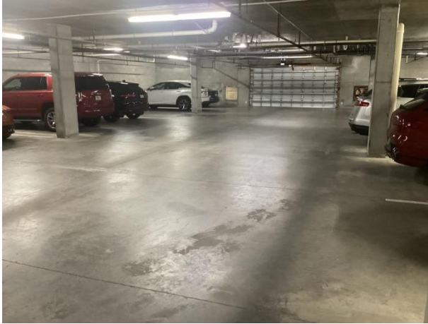
On-grade garage floor overview
