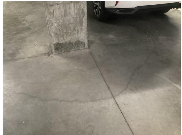
Concrete cracks
