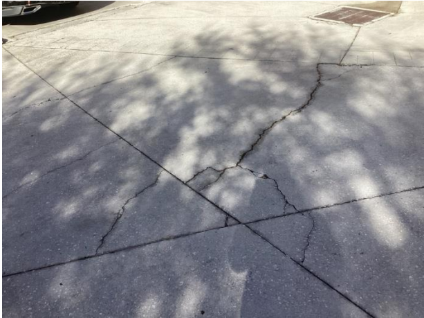
Concrete cracks
