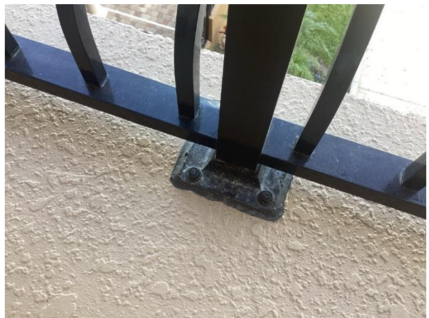
Mechanically attached railing post
