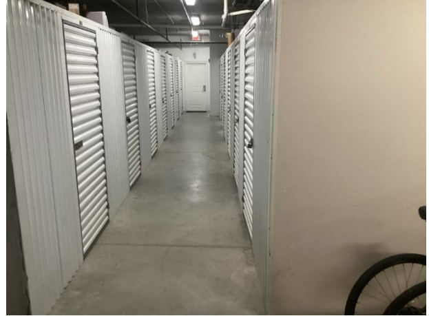
On-grade garage floor overview
