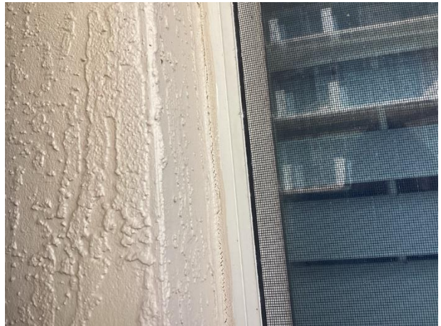
Sealant deterioration
