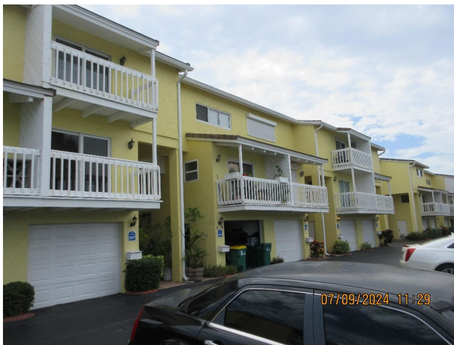
View of west elevation
