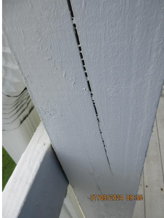
View of splitting wood column
