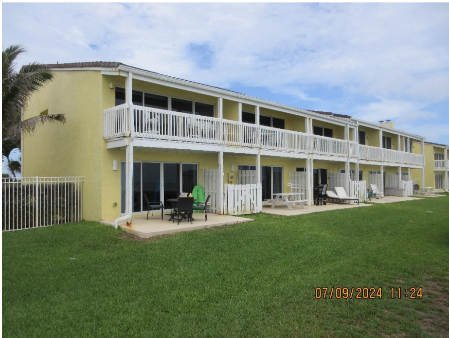
View of Building B east elevation
