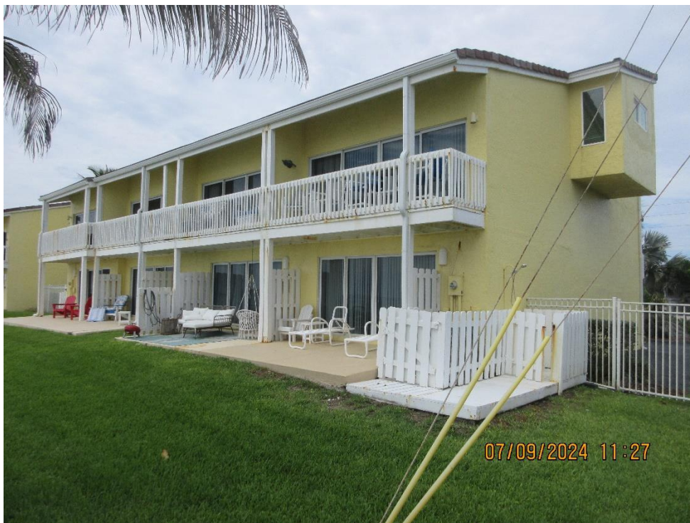
View of Building D east elevation
