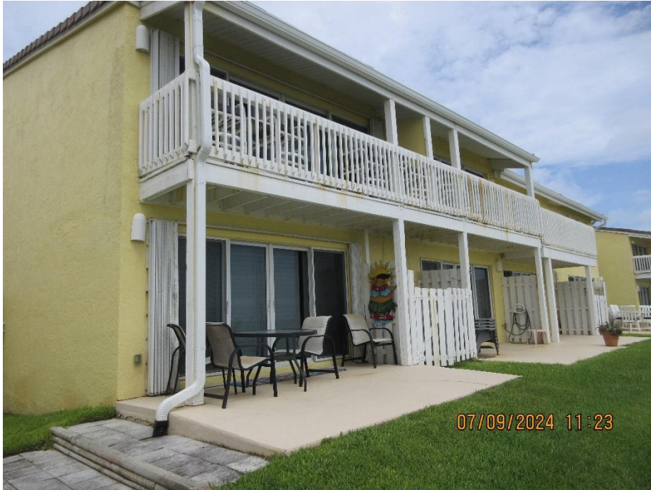
View of Building A east elevation
