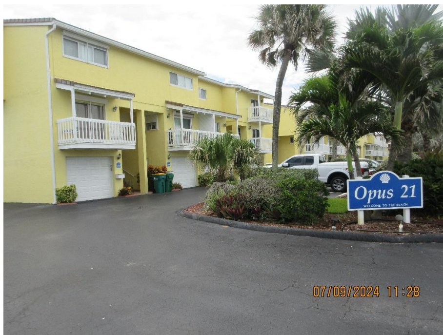
View of west elevation
