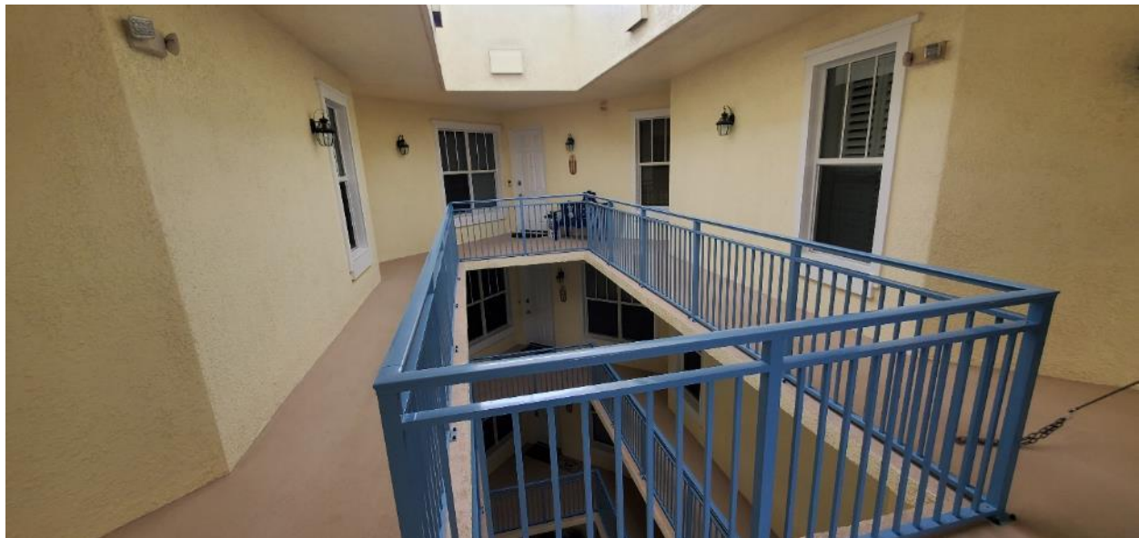
Example of floor coatings on exterior walkways
