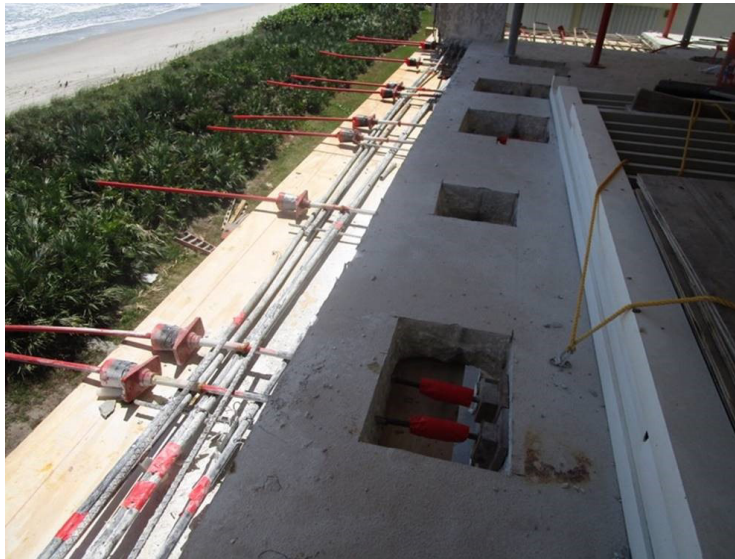
Balcony Slab Edge Repairs with PT Cables Example
