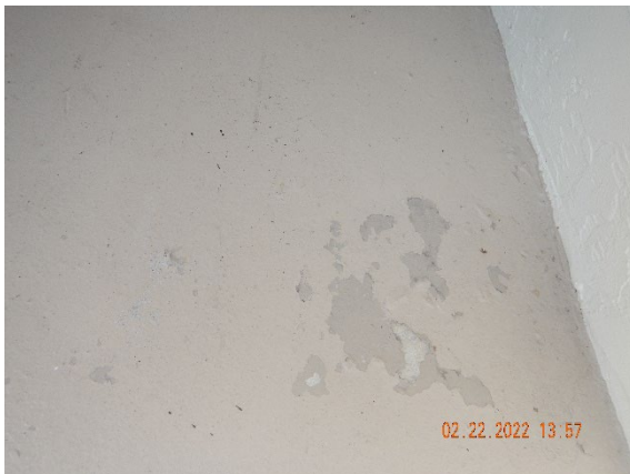
Photograph 9: Chipped textured acrylic coating
