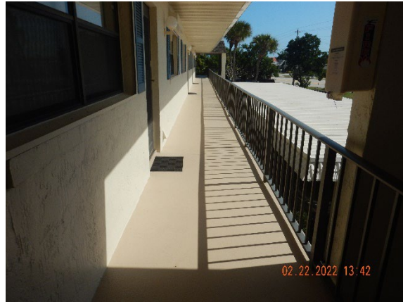
Photograph 6: Typical walkway guardrail
