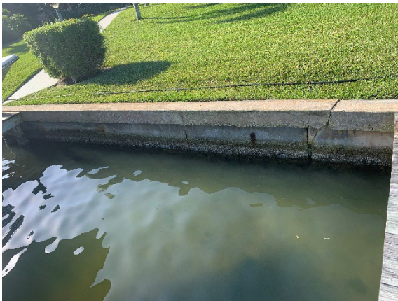
Photograph 15: Seawall panel and cap
