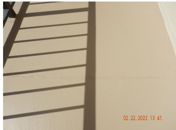
Photograph 10: Coating with very little texture
