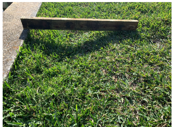
Photograph 16: Different location washout
