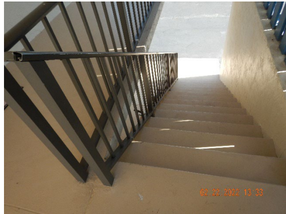
Photograph 2: Typical stairway railing
