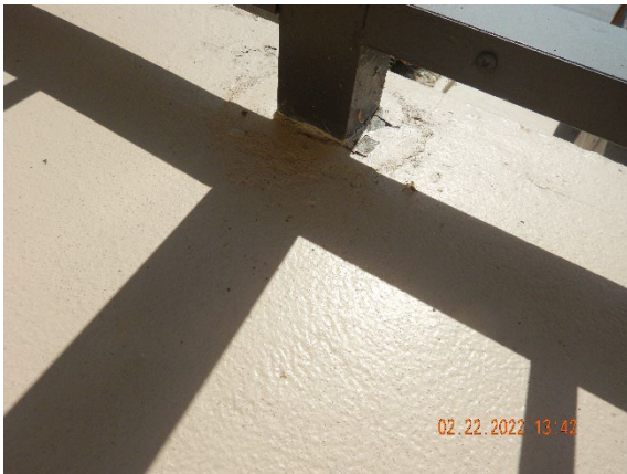
Photograph 3: Embedded post pocket
