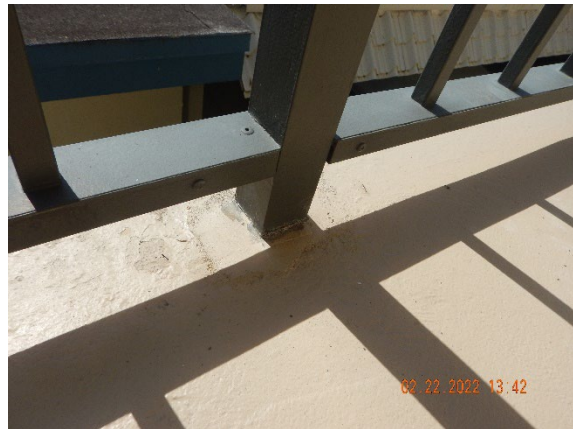
Photograph 8: Embedded rail post
