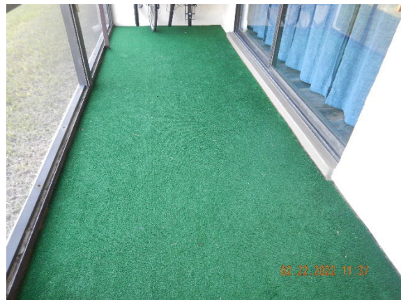
Photograph 12: 4 Carpet on the deck
