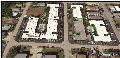
311 Taylor Roof Cover
