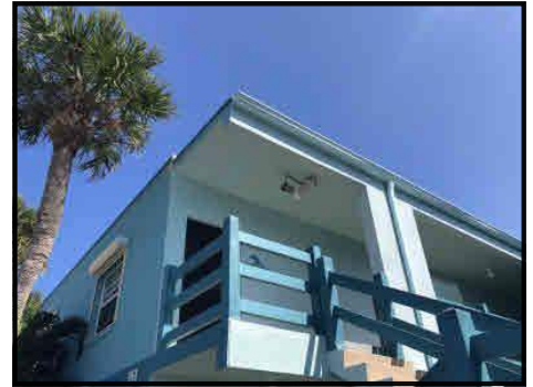
Concrete Roof Deck
