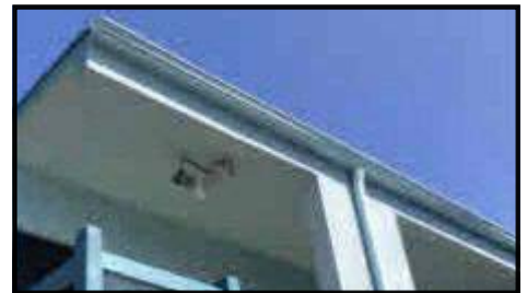
311 Taylor Concrete Roof
