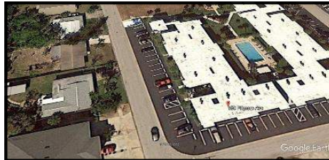
350 Fillmore Roof Cover
