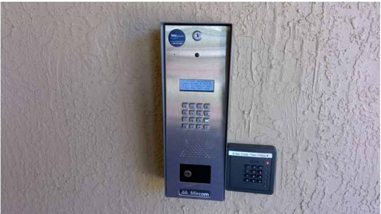
Access Control - Enterphone Panel
