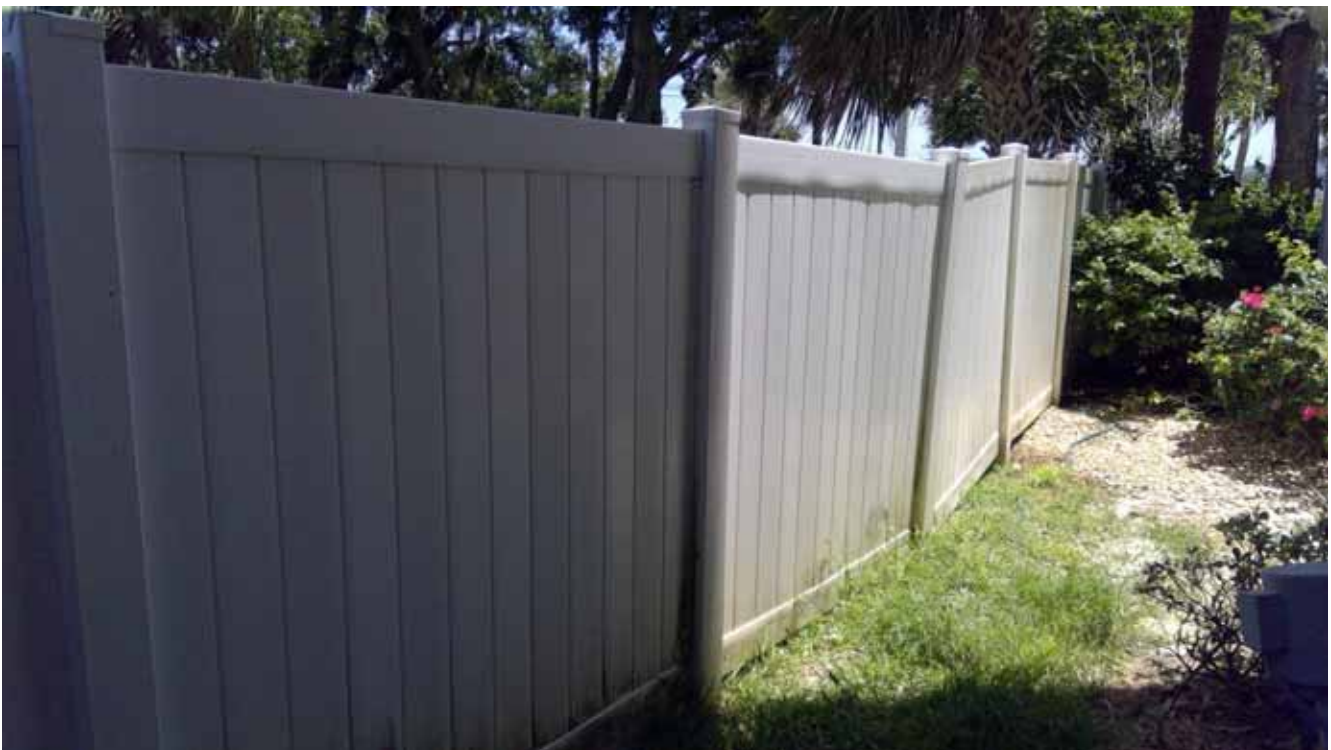
Fence - North Property Line
