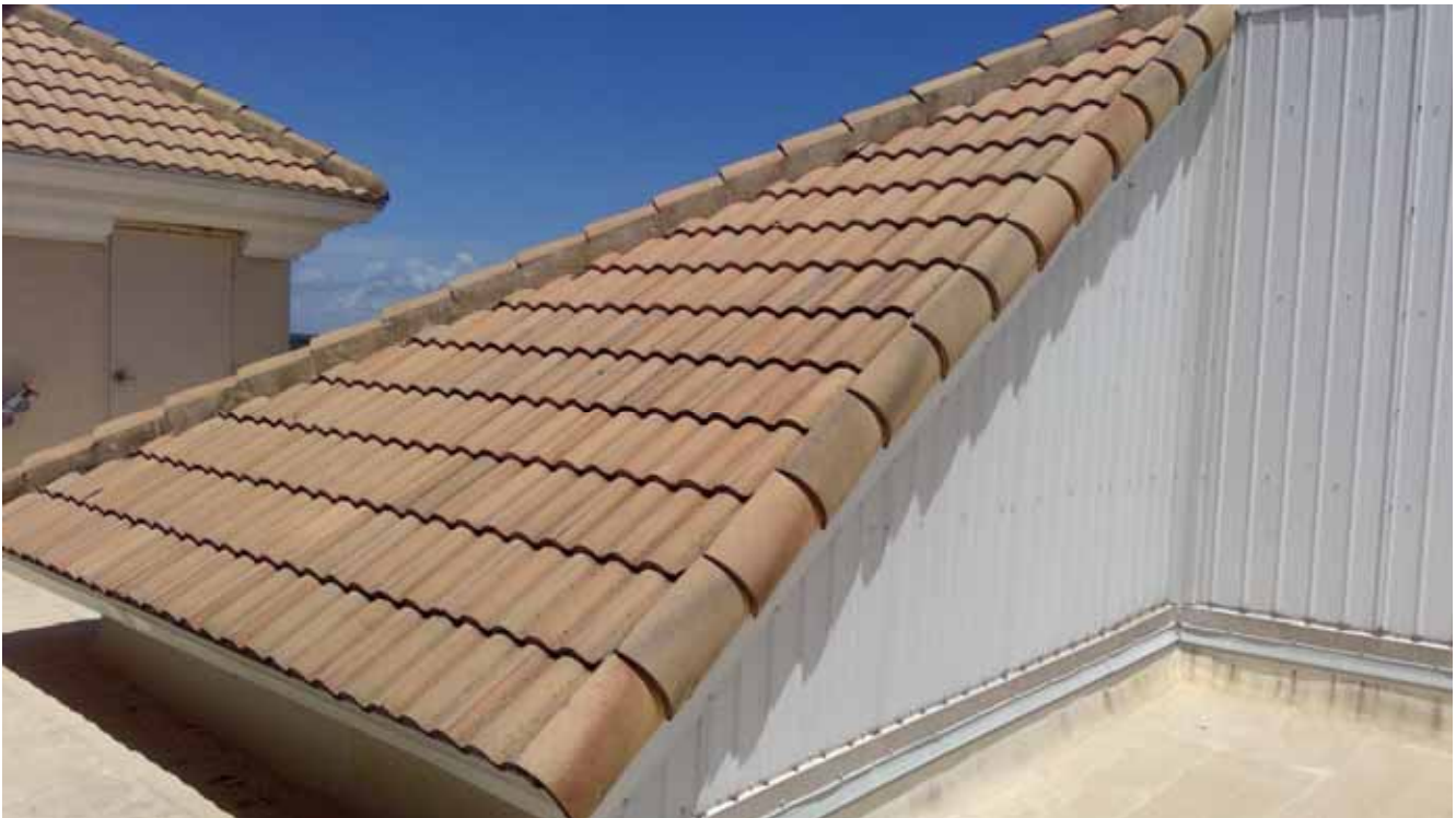
Roof, Concrete Barrel Tile
