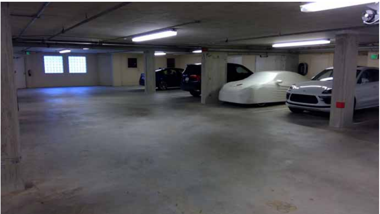
Parking Garage - Level 1
