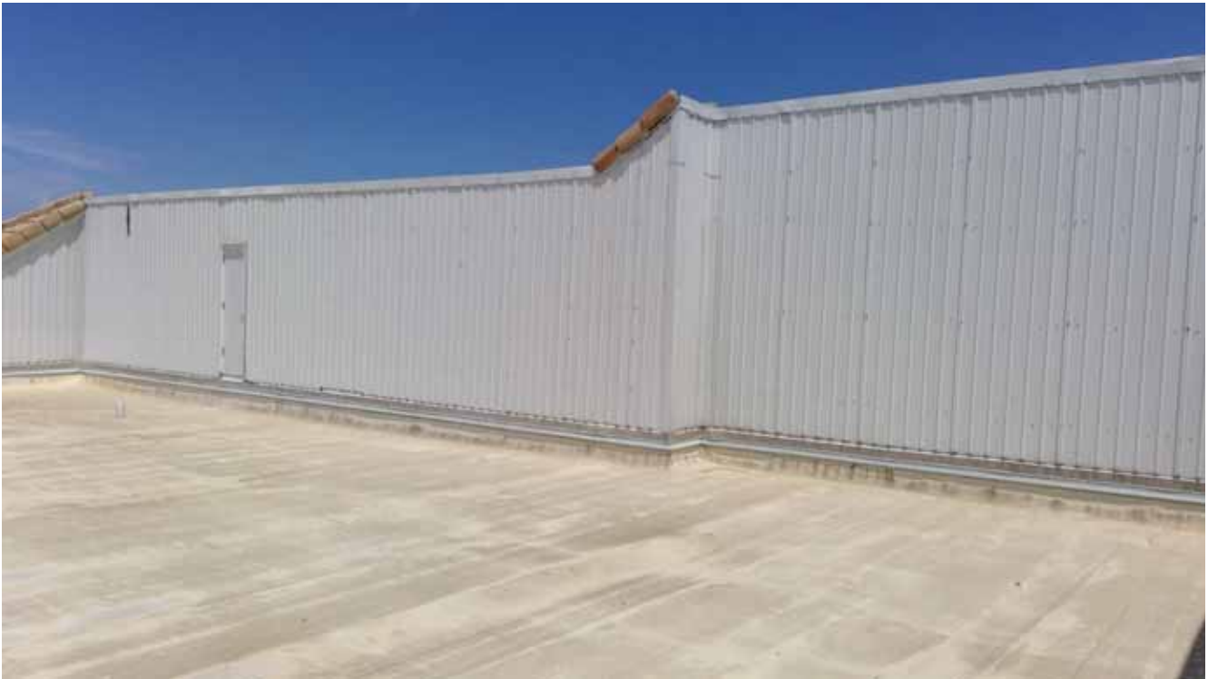
Metal Siding - Roof Parapet Wall
