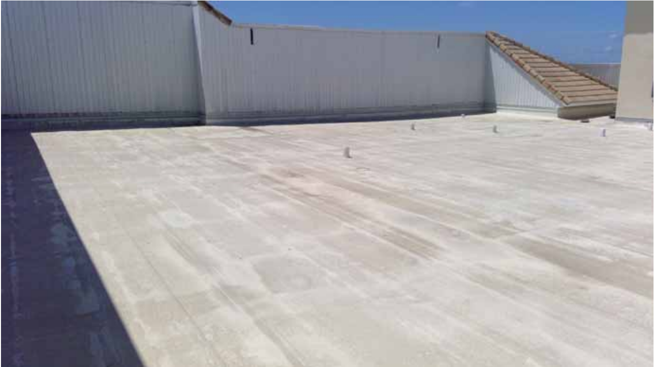
Roof, Modified Membrane
