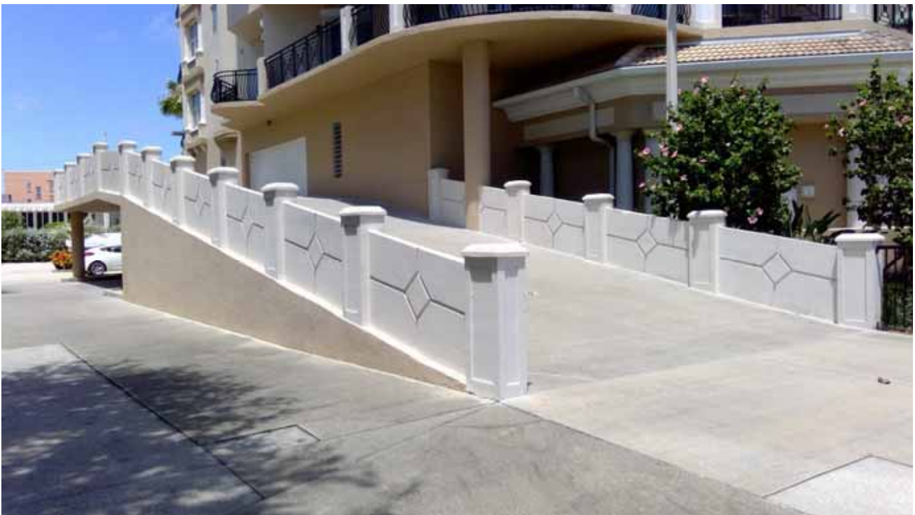
Parking Garage Access, Ramp
