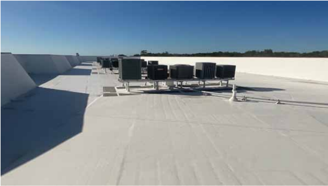
North Condo Bldg Roof
