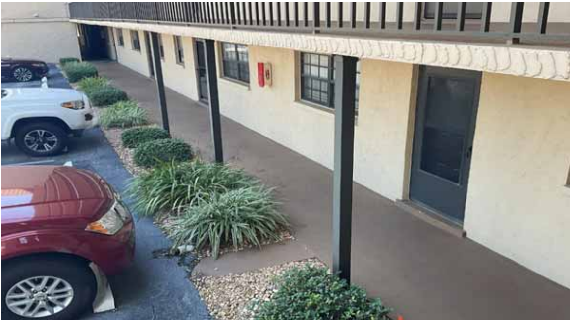
South Condo Bldg Support Posts
