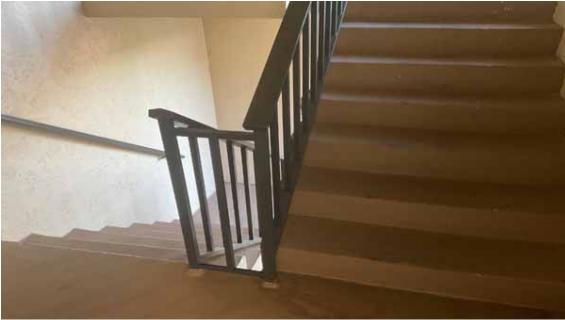
North Condo Bldg Stairwell
