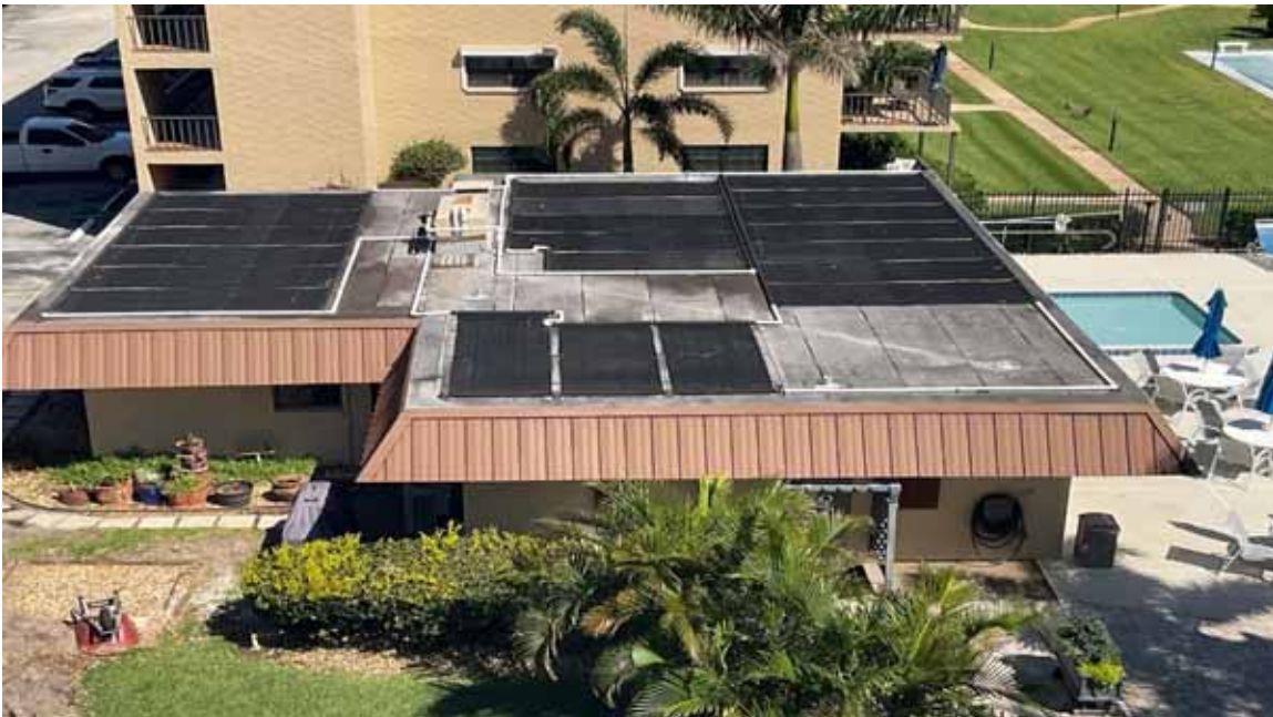
Pool House Bldg Roof & Pool Solar Panels
