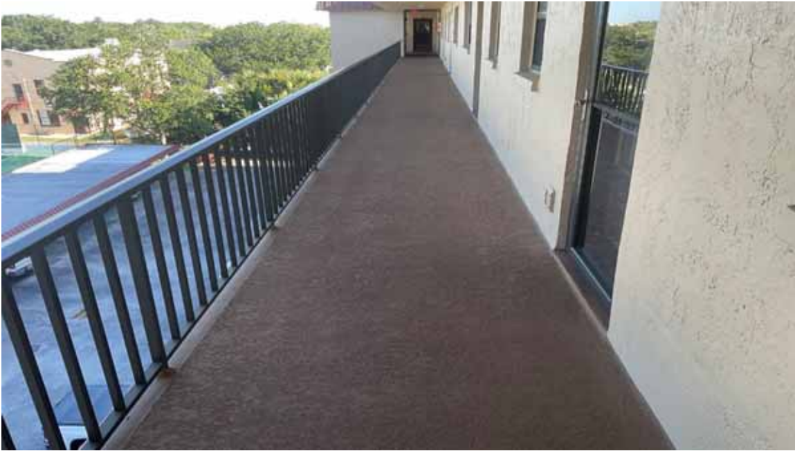
North Condo Bldg Common Walkway
