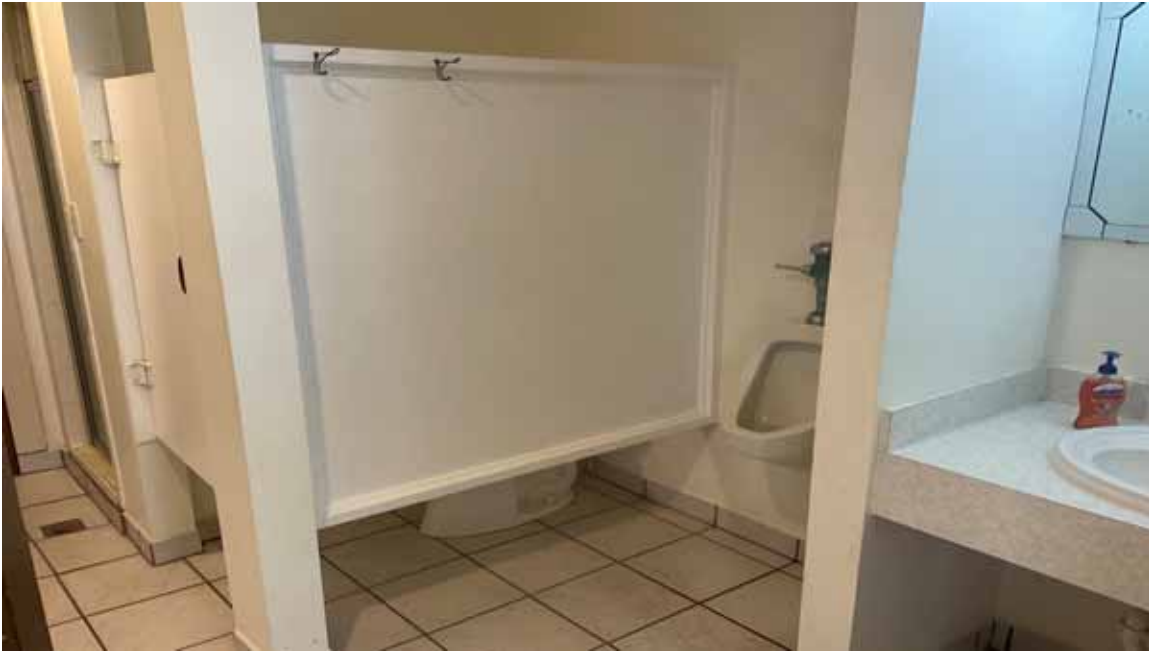
Pool House Bldg Restroom, Men's
