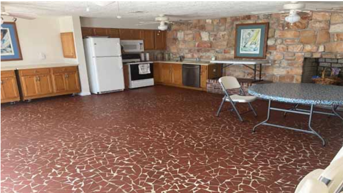
Pool House Bldg Main Room
