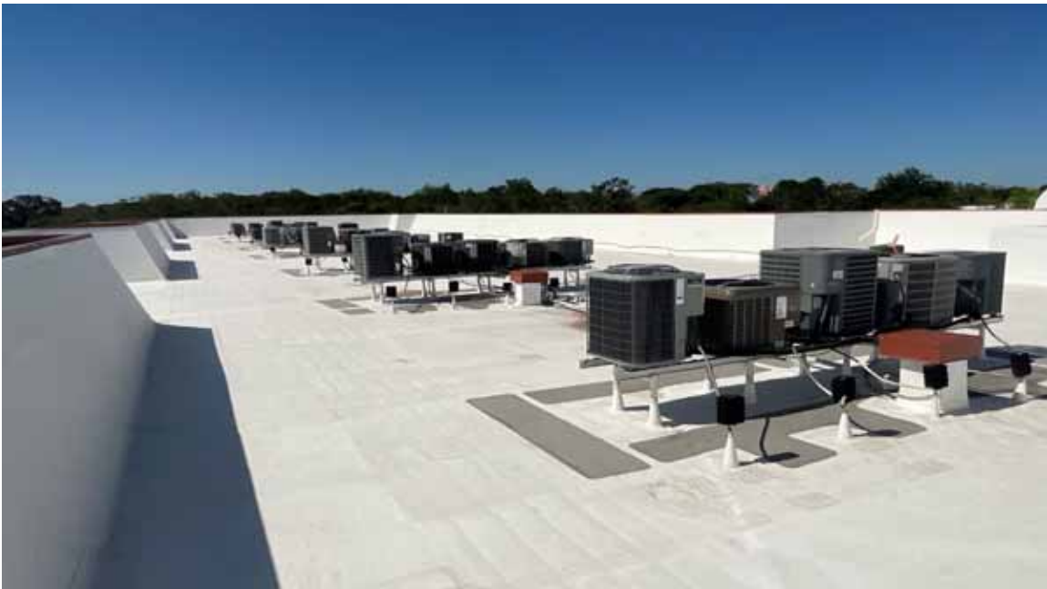
South Condo Bldg Roof
