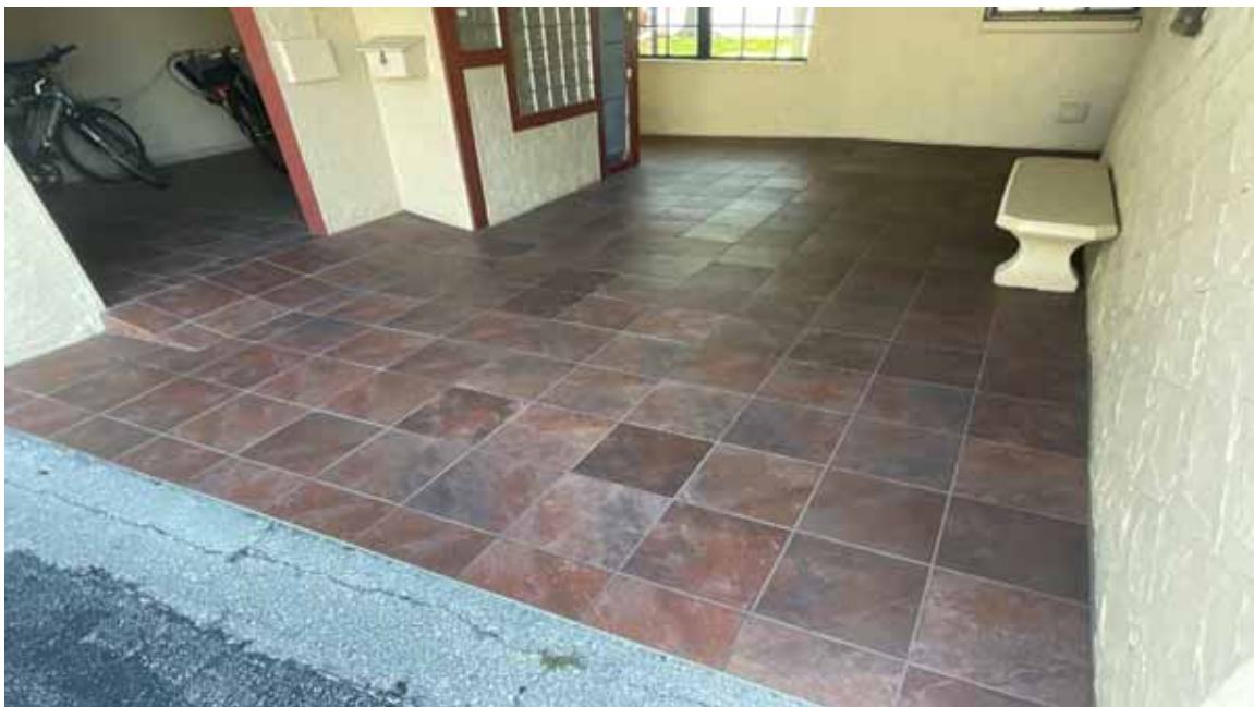
South Condo Bldg Lobby Tile
