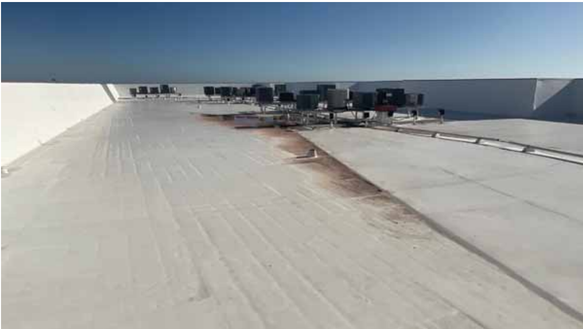
North Condo Bldg Roof
