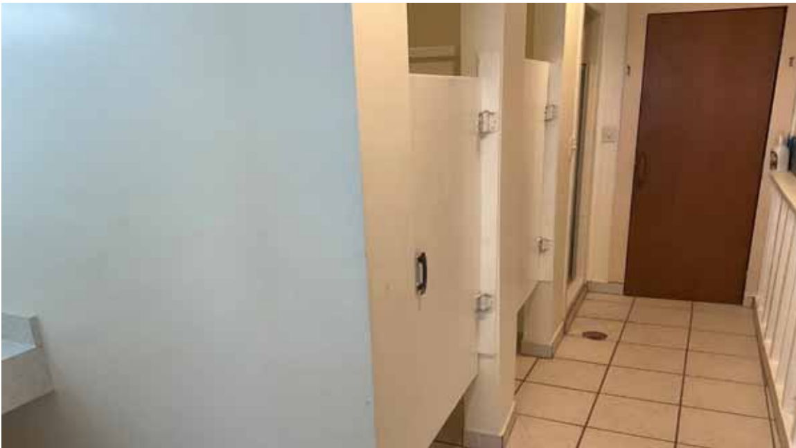
Pool House Bldg Restroom, Women's
