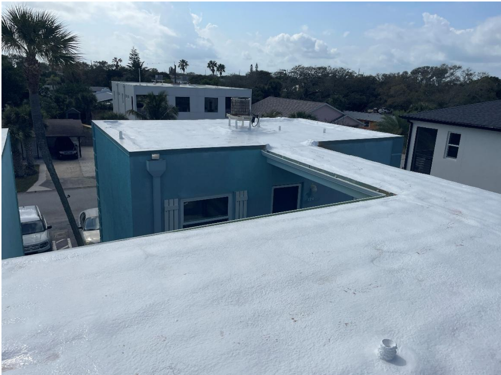
Photos of the newly installed Spray Polyurethane Foam roof system with silicone coating.
