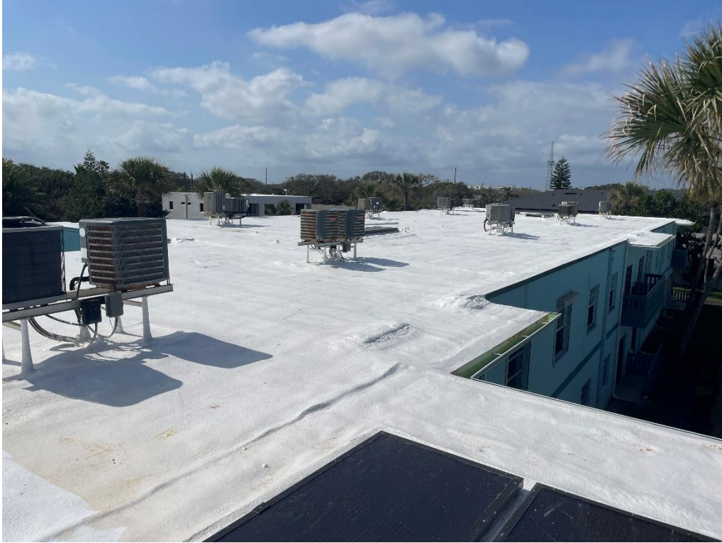
Photos of the newly installed Spray Polyurethane Foam roof system with silicone coating.
