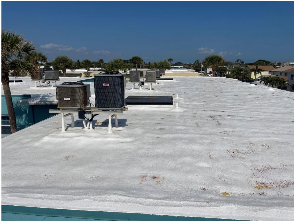
Photos of the newly installed Spray Polyurethane Foam roof system with silicone coating and new skylights.
