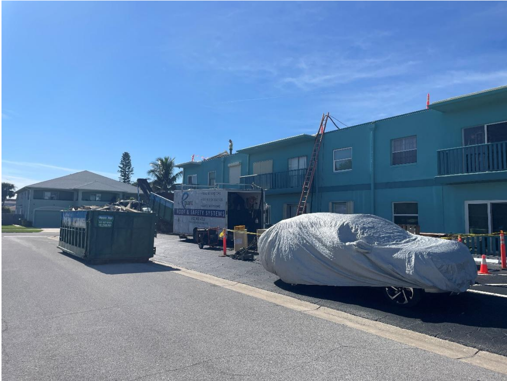
Street view of Building F
