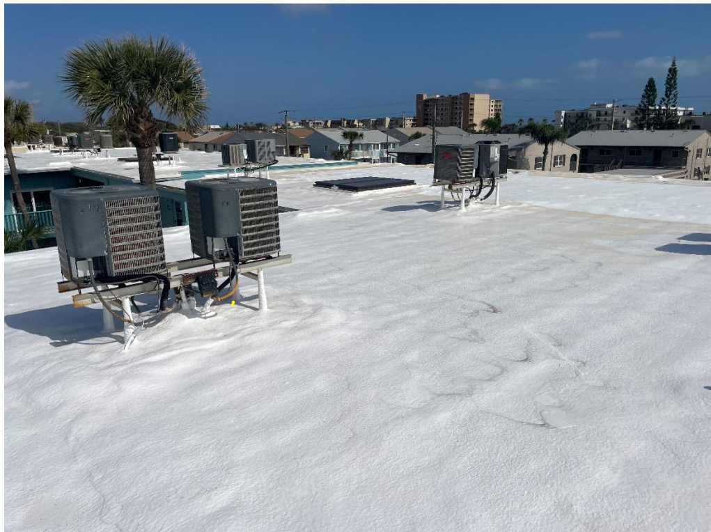
Photos of the newly installed Spray Polyurethane Foam roof system with silicone coating and new skylights.
