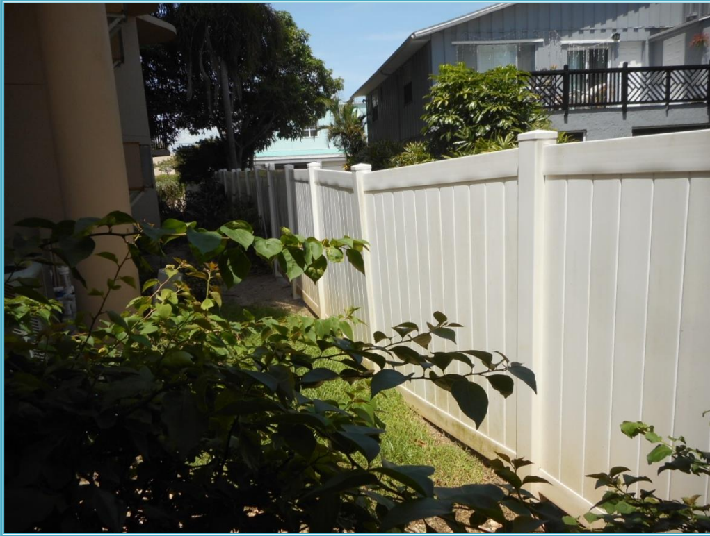
VINYL FENCE ALONG NORTH PERIMETER
