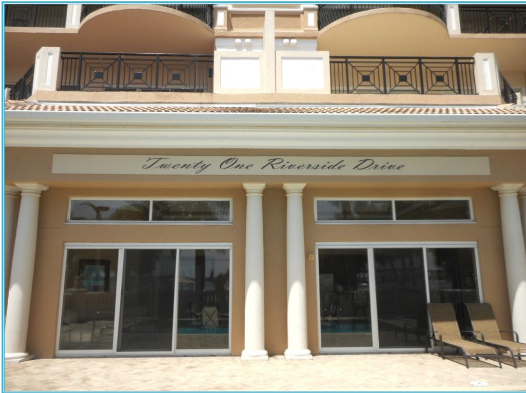
EAST ELEVATION, GROUND LEVEL
