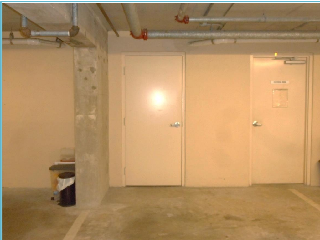
STORAGE UNITS IN PARKING GARAGE
