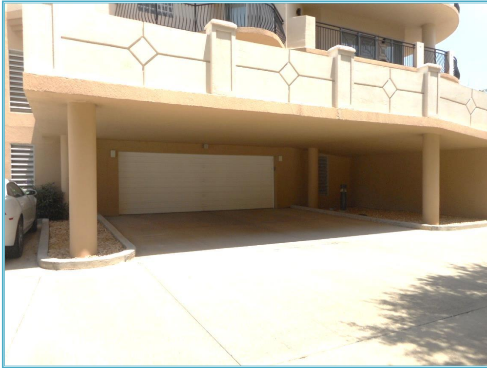
ENTRANCE TO FIRST LEVEL PARKING GARAGE
