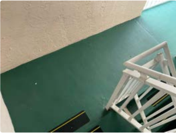
Typical stair landing
