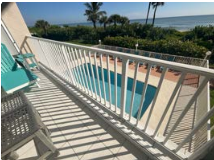
Typical balcony railings
