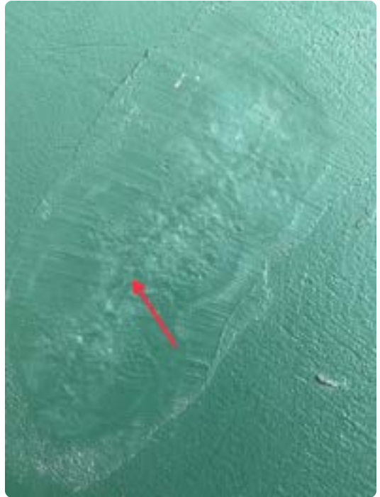
Hollow area near Unit 201. Has had previous remediation and is currently cracking.
