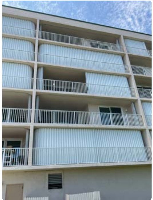
Typical middle balcony stack
