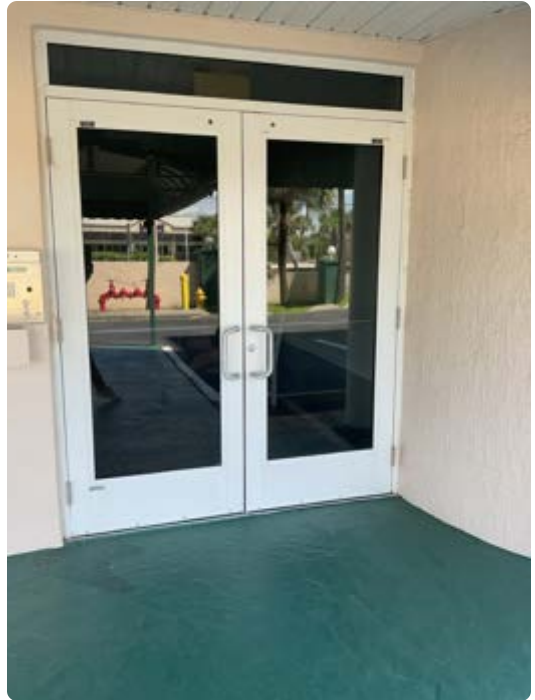
Front entry storefront doors
