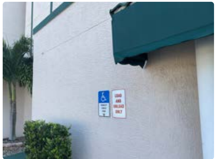
Typical exterior wall paint
