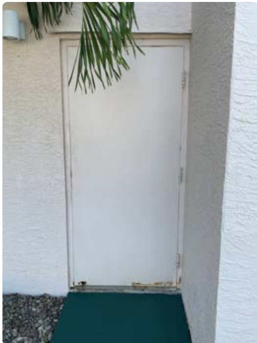
Stairwell exit door
