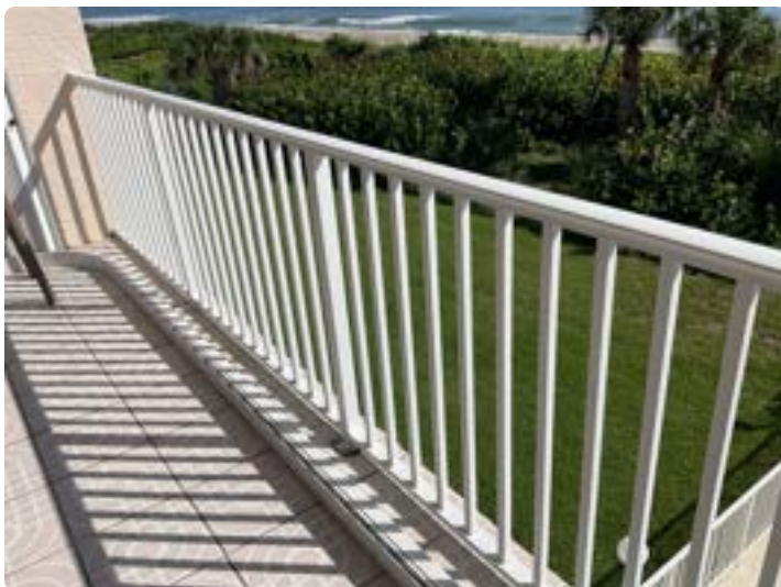
Typical balcony railings
