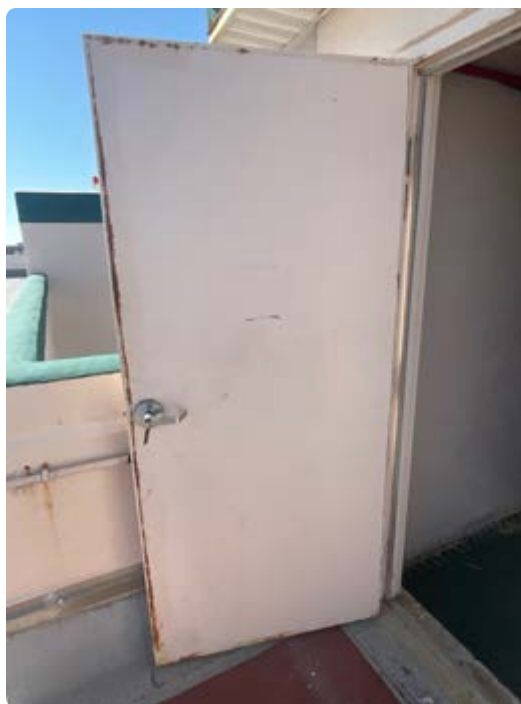
Roof entry door
