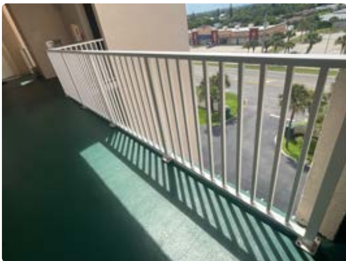
Typical walkway railings
