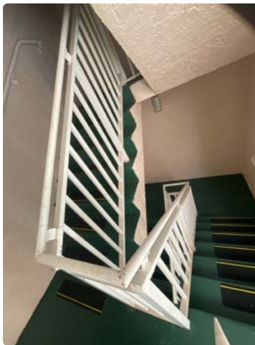
Typical stair railings
