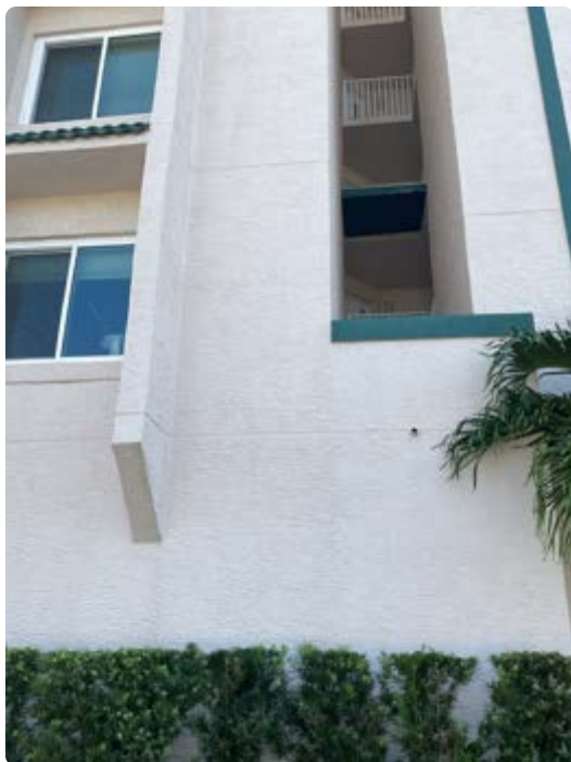
Typical exterior wall paint
