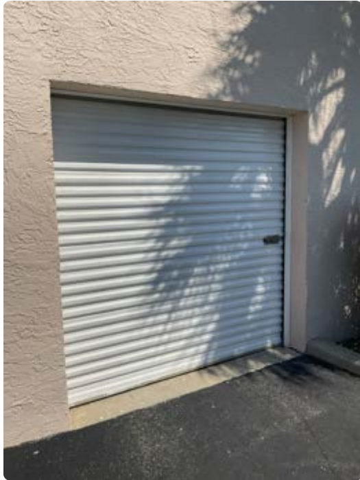
Trash room pull up door
