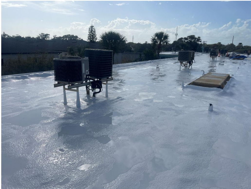
Photos of the newly installed Spray Polyurethane Foam roof with silicone coating.
