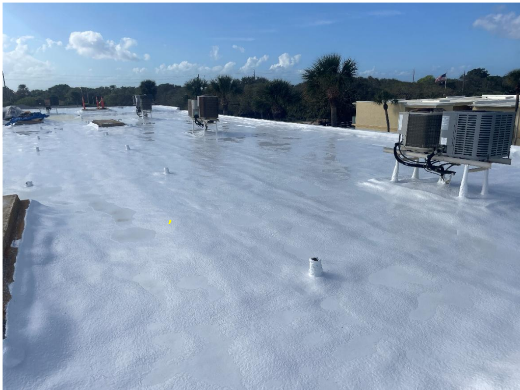
Photos of the newly installed Spray Polyurethane Foam roof with silicone coating.
