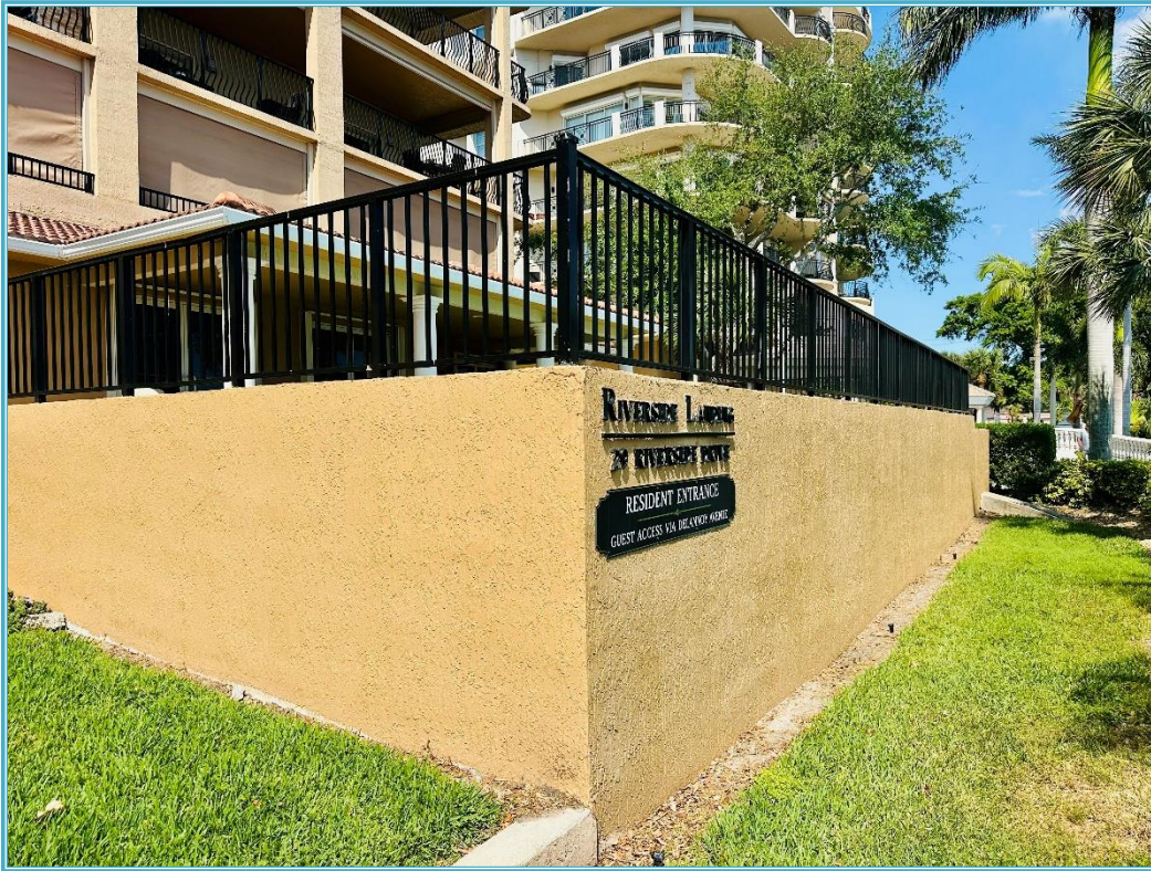
POOL ENCLOSURE AND RETAINING WALL
