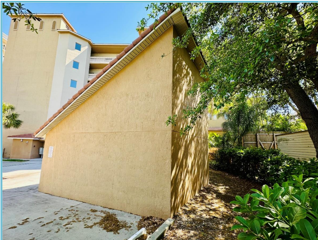
SOUTHWEST CORNER OF ATTACHED GARAGE
