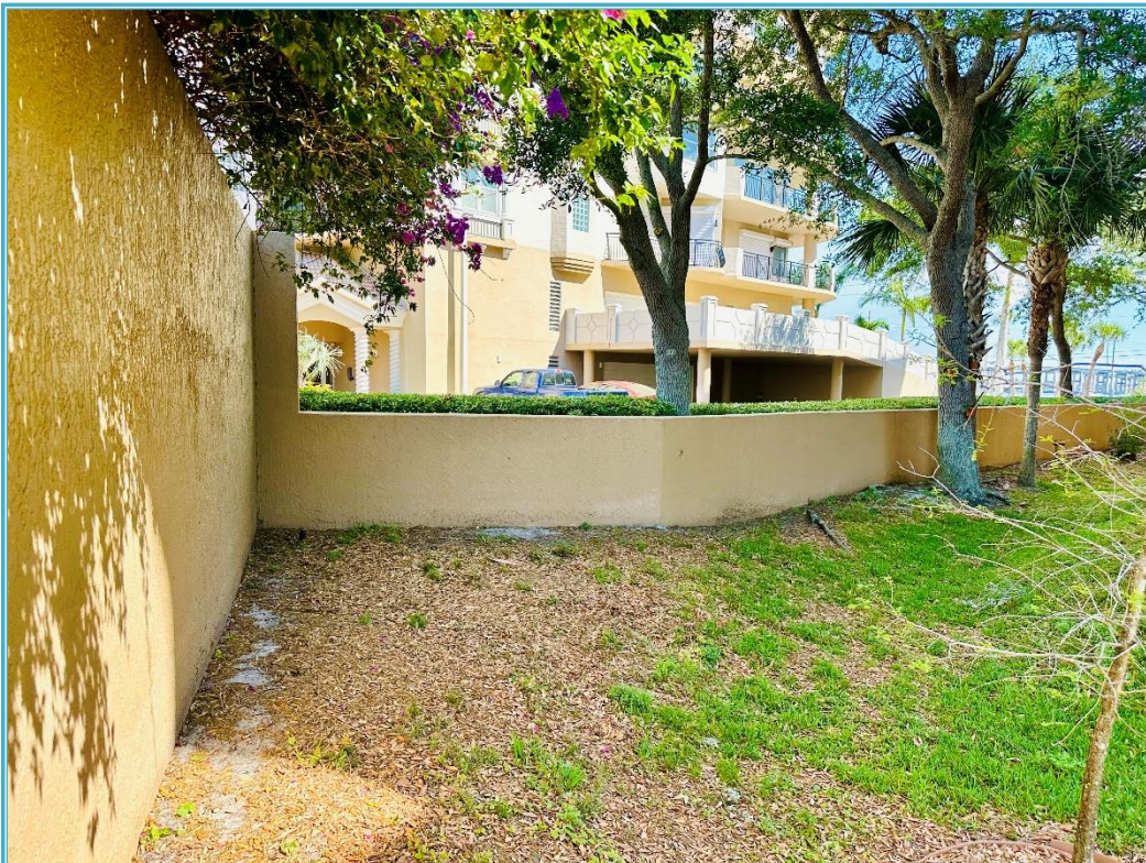
NORTH PERIMETER WALL
